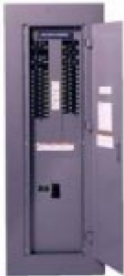
Figure 22: Panelboard (flush wall-mounted).
